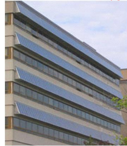
PV overhangs Queen's University (retrofit)
